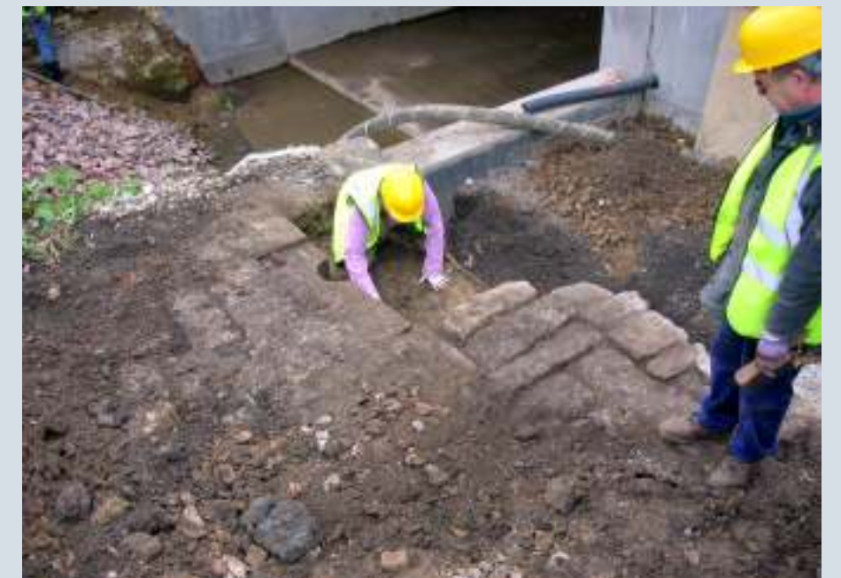
Examining Swing Bridge abutments at Ebley
