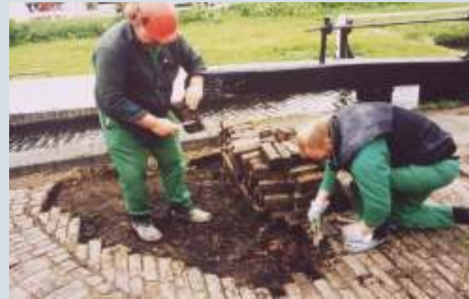
Waterway Training - bricklaying
