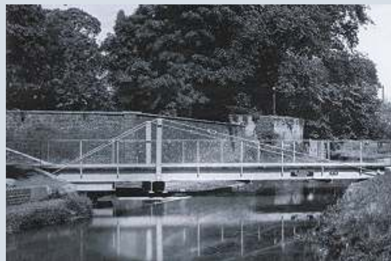
Lodgemore Swing Bridge - 1928 Steel Replacement
