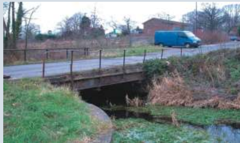
Upper Mills Swing Bridge - remains of the 1928 structure
