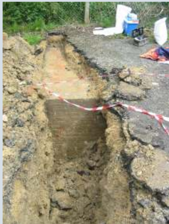
Hope Mill Lock - trial pit exposing former lock wall
