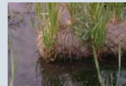
Coir Bank Protection
