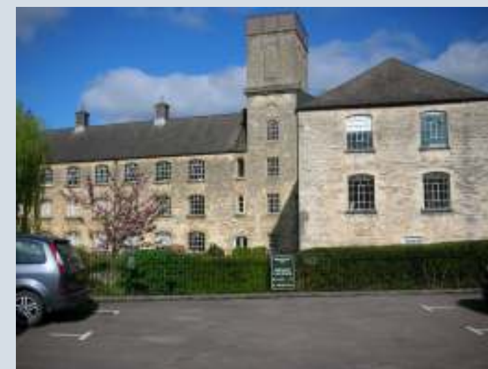
Brimscombe Port Mill - east face overlooking the Port
