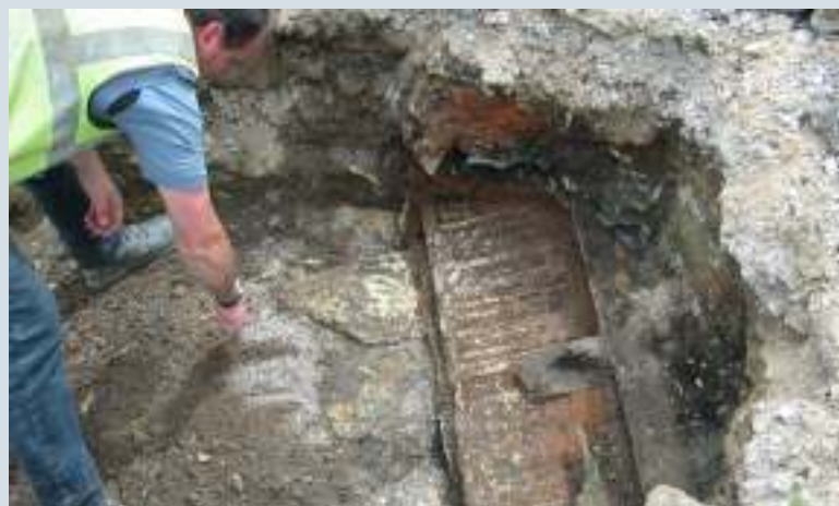
Brimscombe Port - trial pit showing edge of narrowboat dock
