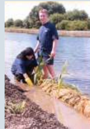
Bank Protection - Coir Roll / Hazelfaggot
