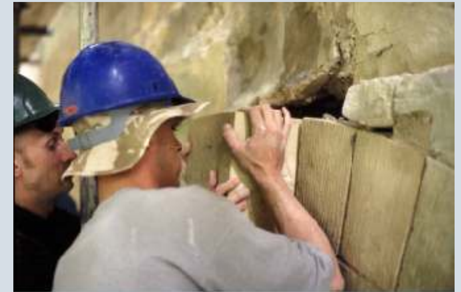
Masonry Training - fitting an arch keystone
