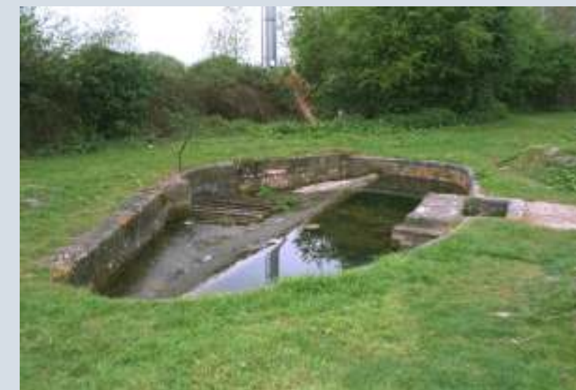
Meadow's Mill Spill Weir
