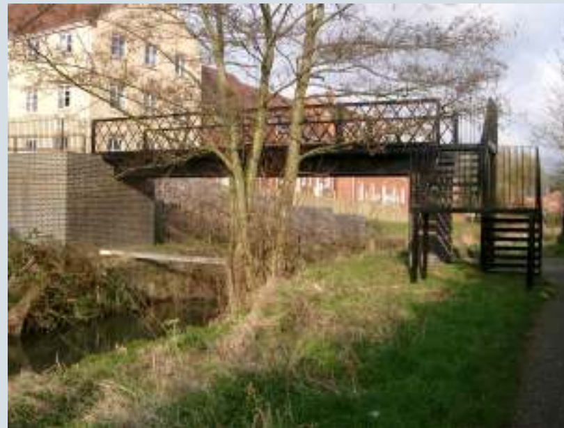
Hilly Orchard Bridge - shows narrowed canal and need for ramped access
