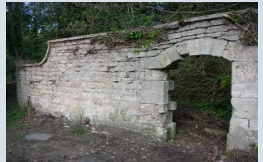
Brimscombe Port - perimeter wall
