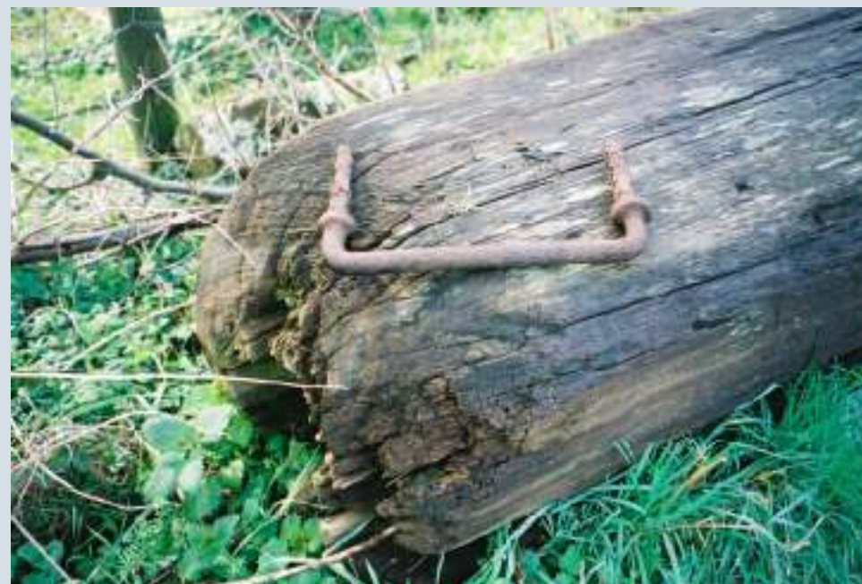
Remains of softwood balance beam at Ryeford Double Lock - with the only surviving handhold staple which spiked into the top of the beam. © David McDougall 2002
