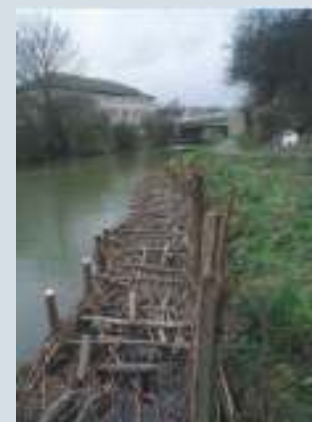
Bank Protection - Coir Roll / Hazelfaggot
