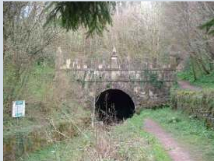
Sapperton Tunnel - Daneway Portal
