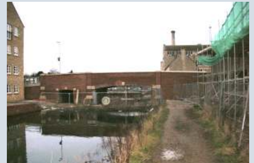
Ebley Road Bridge - constructed without reference to a CMP
