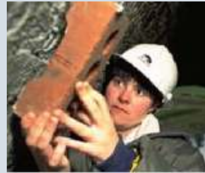
Creating Bat Habitat - introducing a batbrick into a bridge arch
