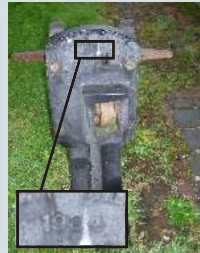
Cast Iron Paddle Stand on Droitwich Barge Canal - with date stamp
