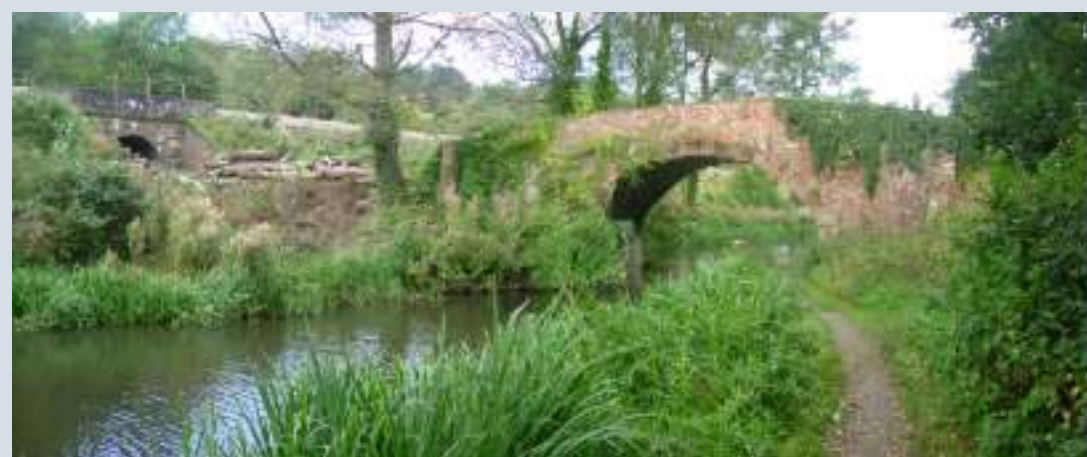
Bagpath Bridge - Thames & Severn section
