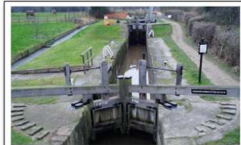
Chesterfield Canal - sympathetic repair of a historic lock
