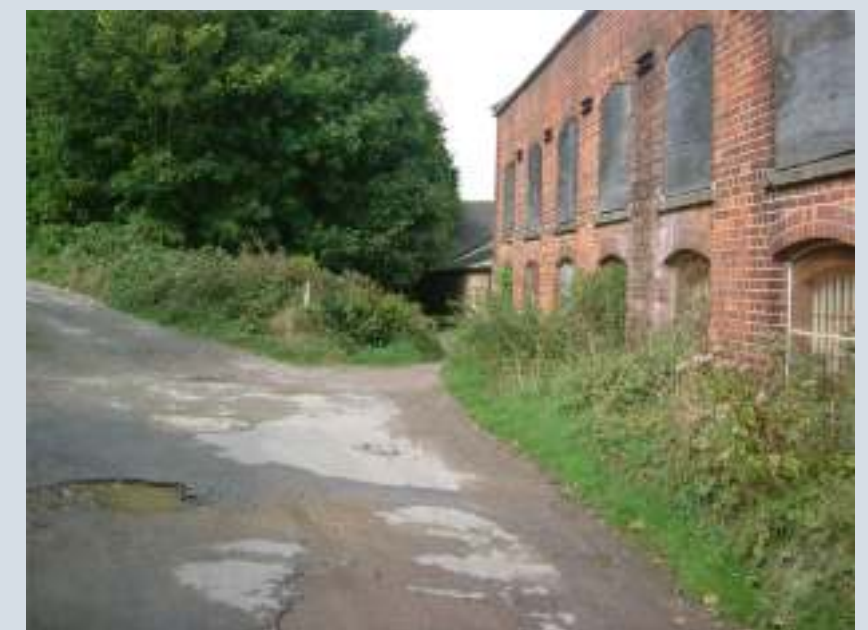
Infilled canal channel
