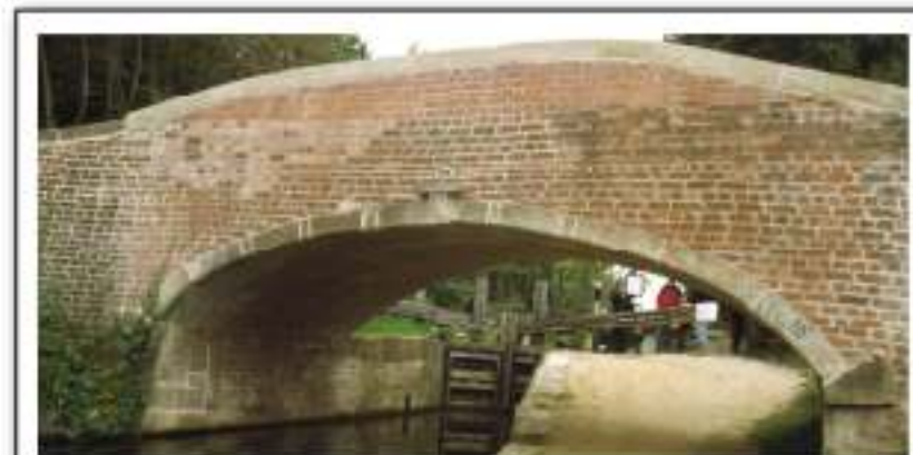
Chesterfield Canal - sympathetic restoration of an historic bridge
