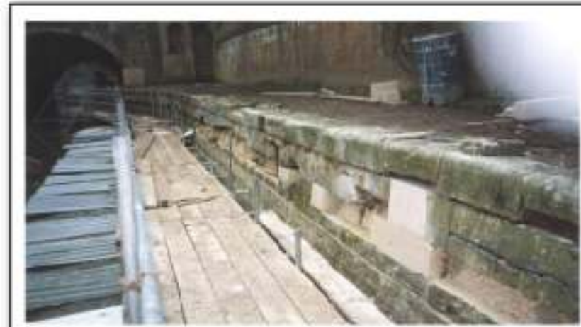
Kennet & Avon Canal - sympathetic repair of wharf wall with new stone
