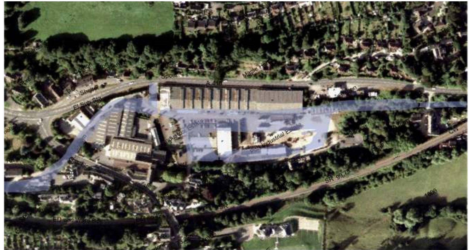
Aerial View of Brimscombe Port - overlay showing shape of original port
