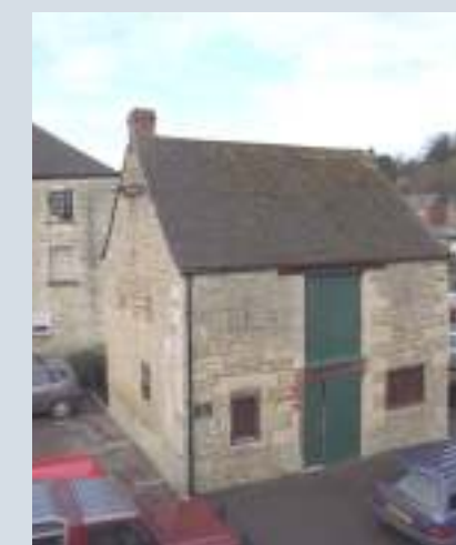
Salt Warehouse - a remnant of the Brimscombe Port Buildings
