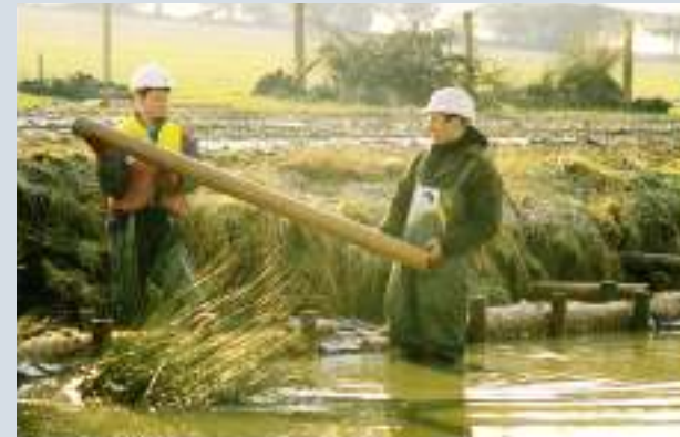
Vole Pipe Laying
