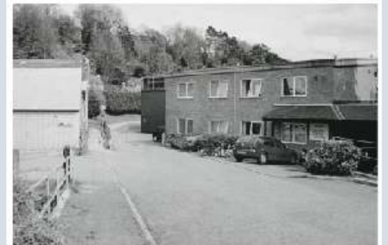
Approach channel today - forming access road
