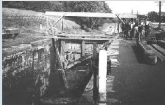
Ryeford Double Lock - Historic gate replacement work
