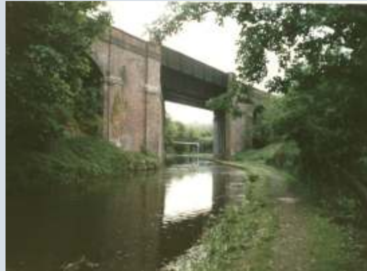
Capel Mill Rail Viaduct - before (1986) construction of bypass
