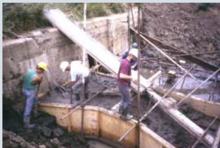
Whitminster Lock - volunteers at work on the new top gates
