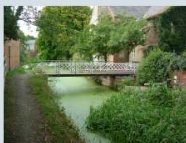
Ryeford Swing Bridge - restored by CCT volunteers
