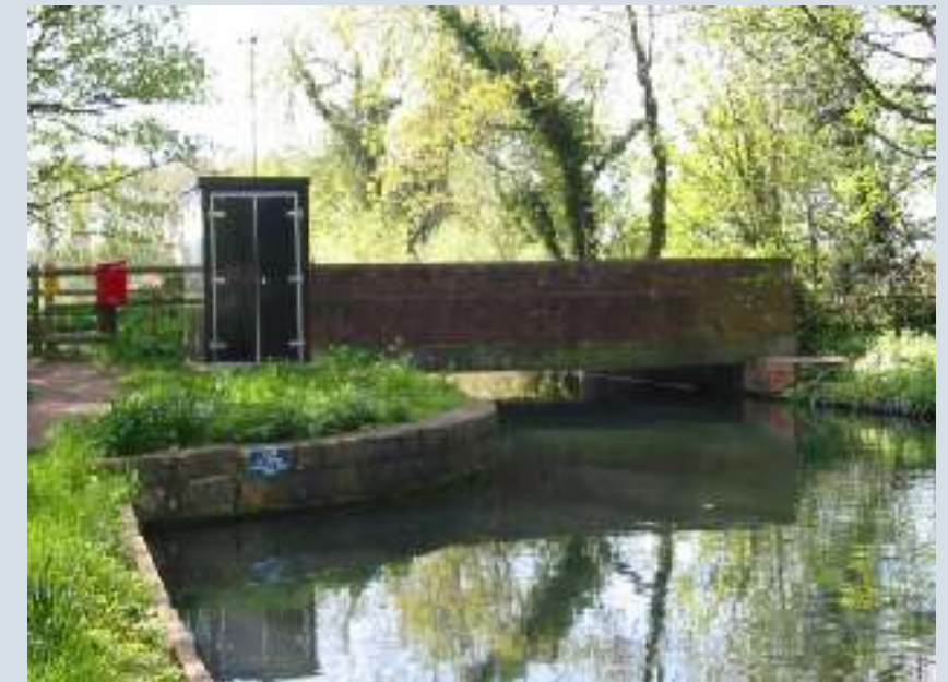
Low Bridge - and obstruction to line of canal
